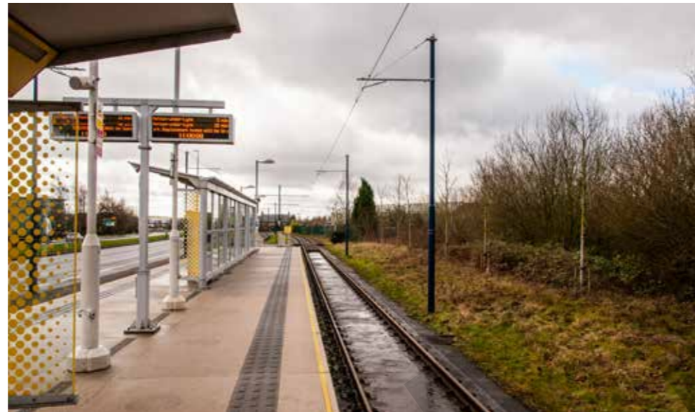
View south west past Ashton Moss Metrolink station
