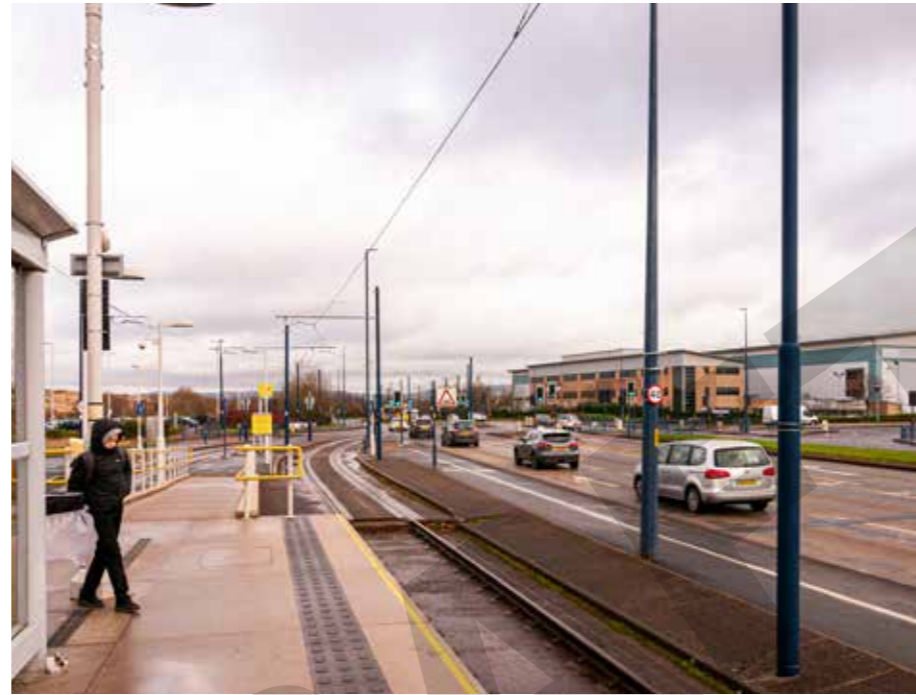
View from Ashton Moss Metrolink station looking north along Lord Sheldon Way
